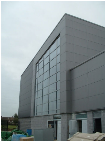
External View Oaklands Pool
